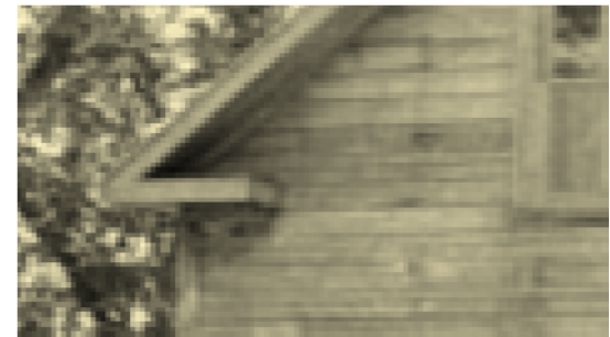
Figure 22. Farm house in the St. Francois-Xavier area. Detail showing the roof return detail suggestive of French flared roofs.
